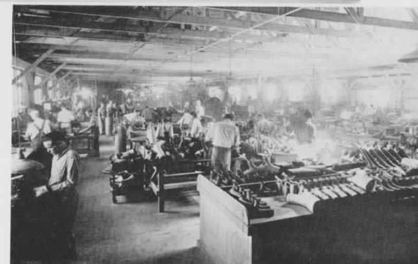
PRODUCTION IN 1936 still centered in Bldg. 1's 50 x 200 ft. shop.
