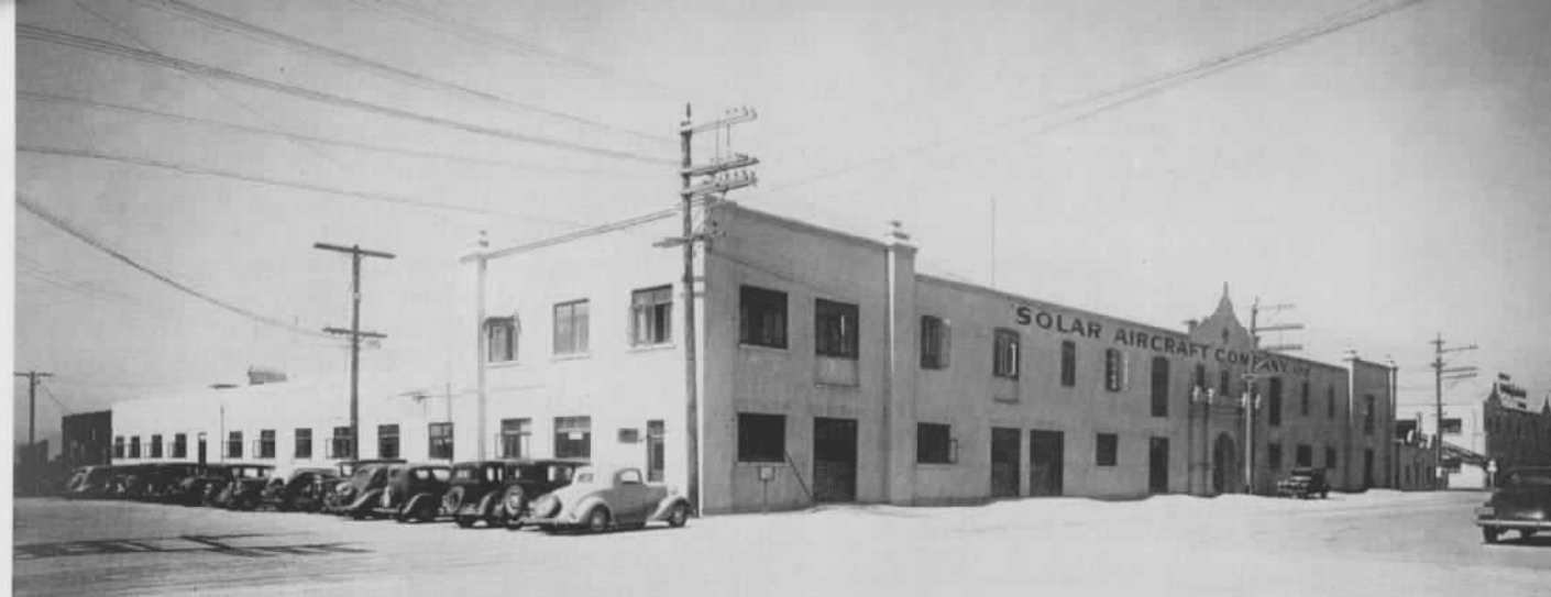
ORDERS CLIMBED—and so did Solar. By 1936 the company had expanded from 1-story Bldg. 1 on Juniper into 2-story Bldg. 2, leased for 15 years.
